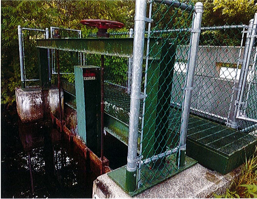
PHOTO 1 VIEW OF DAM FROM UPSTREAM SIDE (ON THE SHORE)
