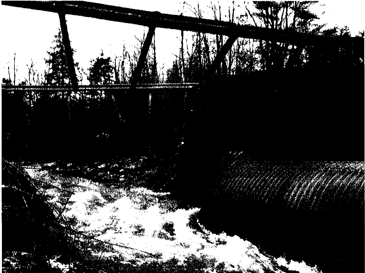
Searles Mill Road Chelsea, culvert washout, April 2007 KCEMA Photo
