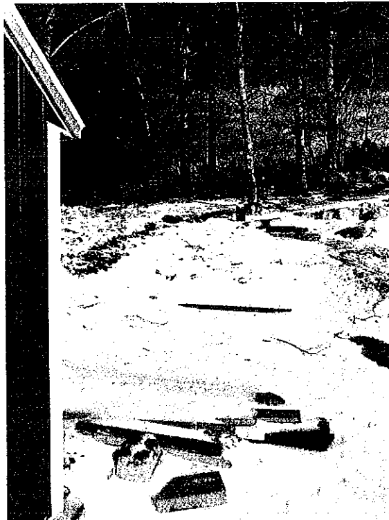
Photo 3: The area immediately behind the new shed, the proposed location to move back to the most practical extent.
