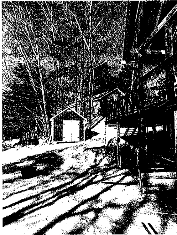
Photo 1: Looking north at the new shed.
