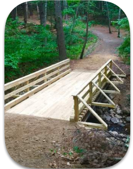
Steel I Beam and PT Bridge
