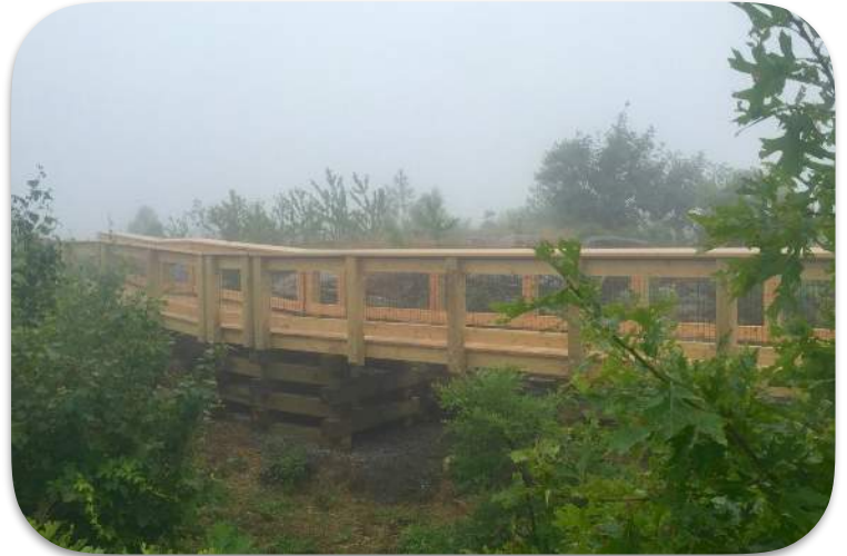
White Oak, Cedar, and Pressure Treated Boardwalk
