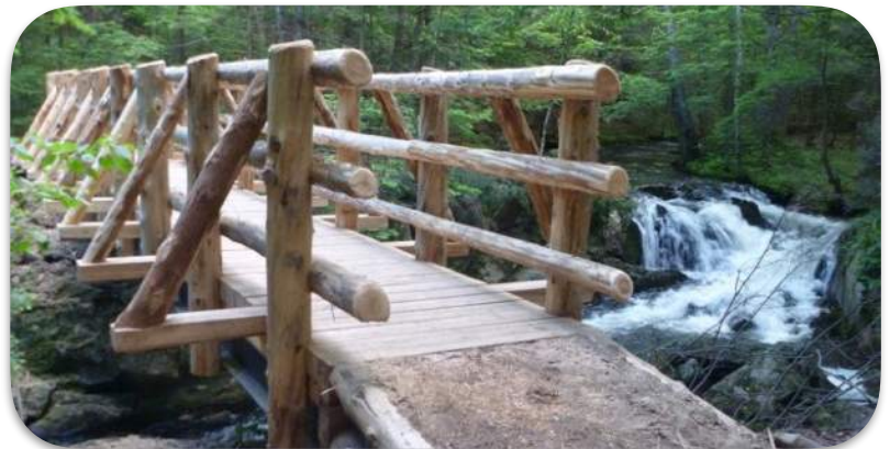
Steel I Beam and Cedar Bridge
