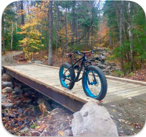
Steel I Beam and Hemlock Bridge
