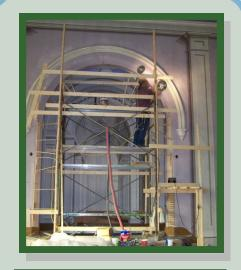
Now that the arch at the front of the Union Meeting House has been jacked up and properly supported from below, the noted decorative painting conservator Tony Castro has removed pieces of broken plaster, closed up cracks that have developed over the decades, and is starting to in-fill new plaster into the cracks. He will finish by painting the new plaster to match the original wall colors. Mr. Castro is on the staging up by the bright light at 1 o'clock.
