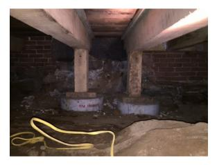
Oak joists supported on piers at main entrance where brick pockets had been removed for granite steps.
